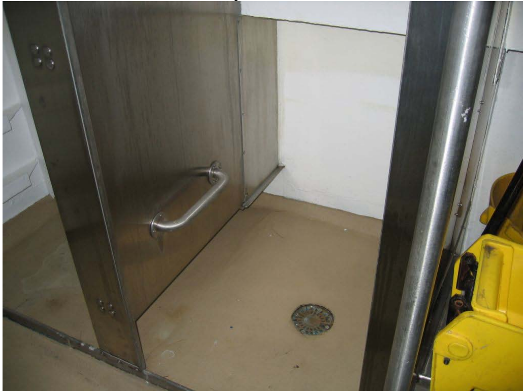
The shower stall decks are in excellent condition
